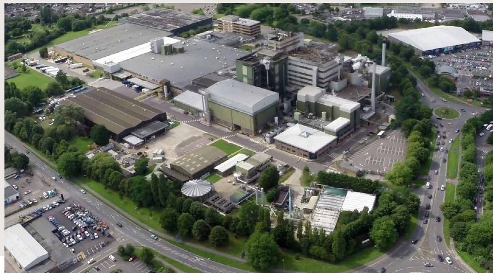
JDE manufacturing facility in Banbury, UK
